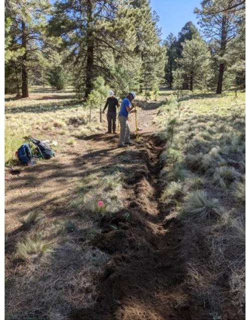
Longer trenches needed to ensure water channeled off the trail stays off.
