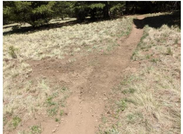
Several small rolling grade dips like this should minimize the effect of water on the cupping process.
